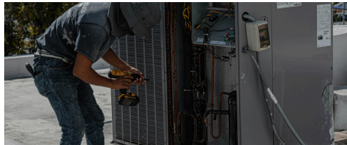
HVAC MECHANICS & INSTALLERS
