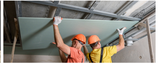
DRYWALL & CEILING TILE INSTALLERS
